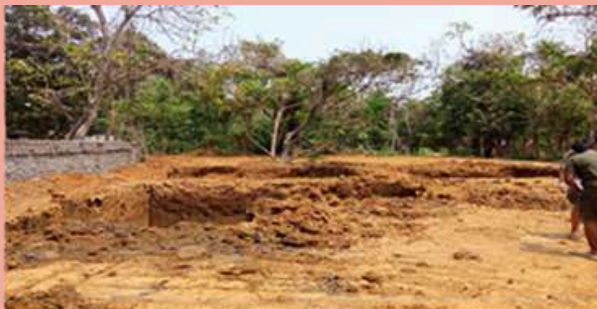
Excavation of land for AS
