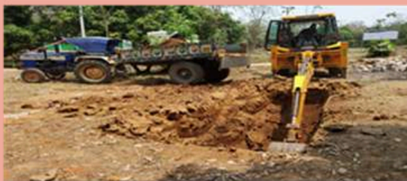
Excavation of land for Chinese Circular hatchery
